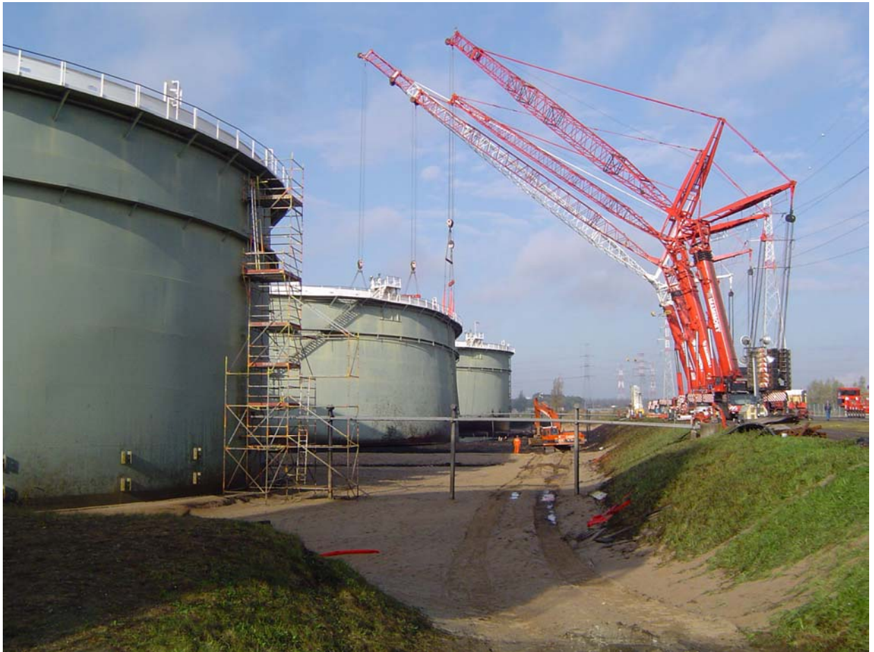
Figure 3: Picture of major cranes stabilising storage tank D2
